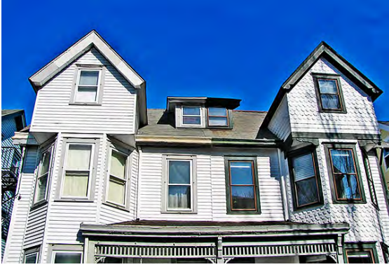
Figure 10. 1. Traditional Duplex with vinyl siding on left and wood siding on the right
