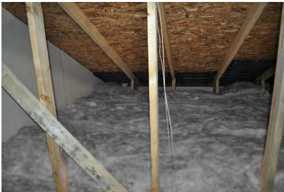
Figure 10. 18. View of vented attic from the attic
