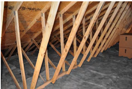
Figure 8. 5: Attic construction
