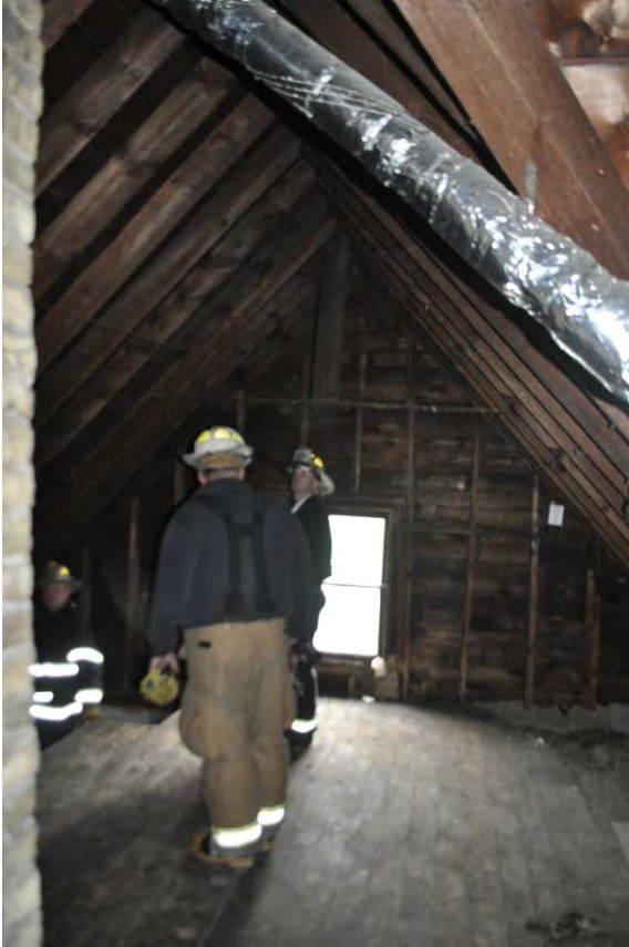
Figure 10. 43: North 9th St attic prior to finishing
