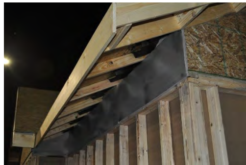
Figure 8. 4: Eave construction detail (before soffit was added)
