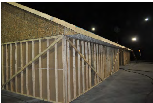
Figure 8. 3: Rear of structure
