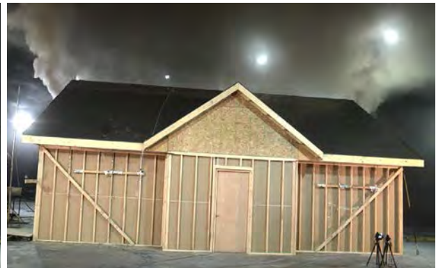
Figure 10.32. Ridge vent after sealing.
