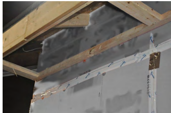
Figure 10. 19. View of unvented attic construction eaves
