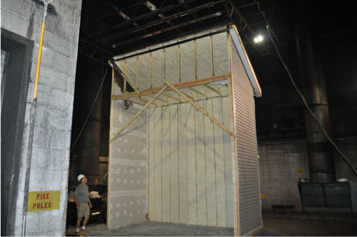
Figure 7. 7: Rear View of Eave Structure for Experiment 3 before drywall application
