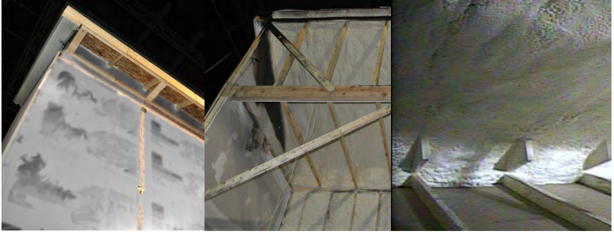
Figure 7. 17: Spray Foam Insulation in Eave Line
