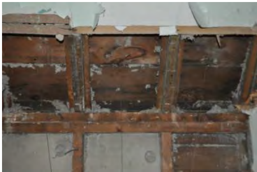
Figure 9. 14: Exp. 1 Ignition Room Wall
