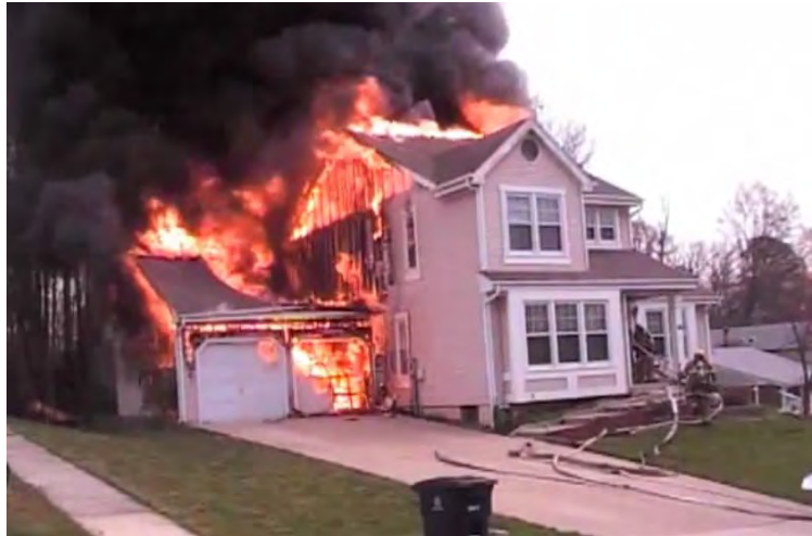
Figure 1. 1: A fire that started in the garage spread up the exterior of the home and into the attic.
