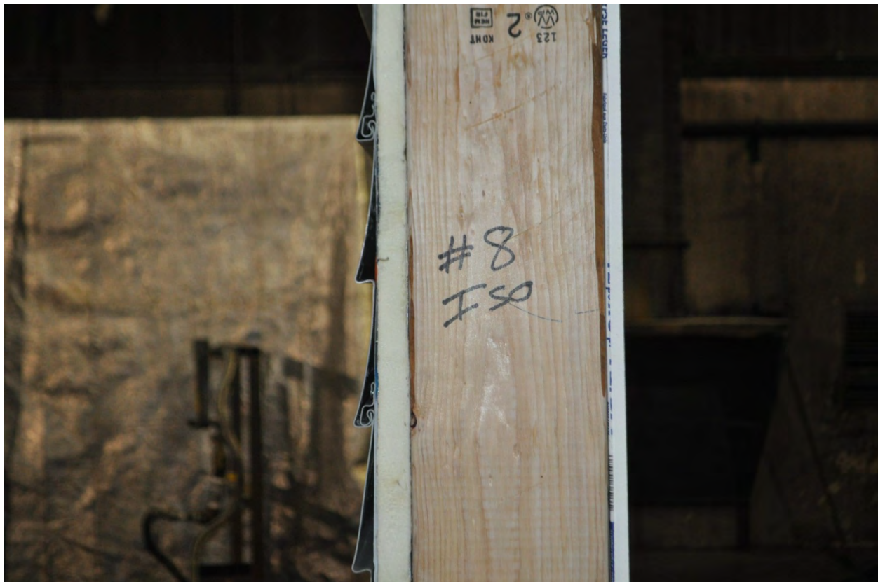
Figure 6. 17: Wall Type 9-I Side View (Side View of 8-I same as Side View of 9-I)
