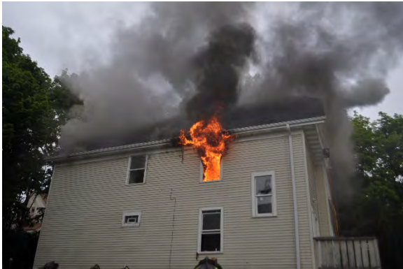
Figure 10. 50. Fire on second floor with extension into the knee wall. Water should be flowed to extinguish the room (from inside or outside) and then flow into the eaves (from inside or outside) before accessing the attic.
