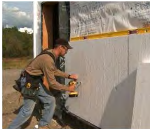
Figure 1. 4: Rigid foam insulation applied to an exterior wall
