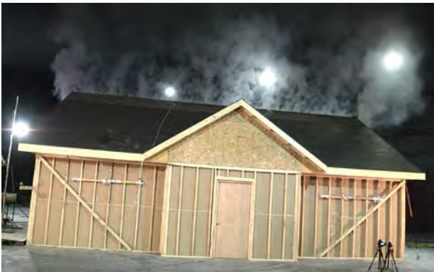
Figure 10.31. Smoke coming from the ridge vent.
