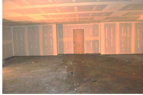
Figure 8. 8: Interior of structure
