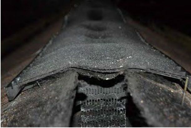
Figure 10. 35. Section cut away after experiment to see ridge vent seal.
