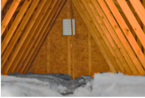
Figure 8. 7: Center of attic and gable vent
