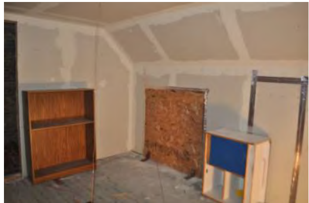
Figure 9. 21: Field Exp. 2 Knee Wall Access Hatch
