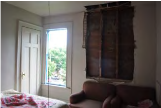
Figure 9. 20: Field Exp. 2 Ignition Room Wall
